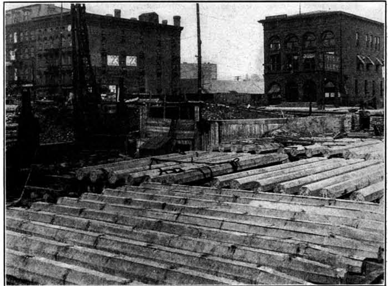
Concrete Piles Cast on the Ground
